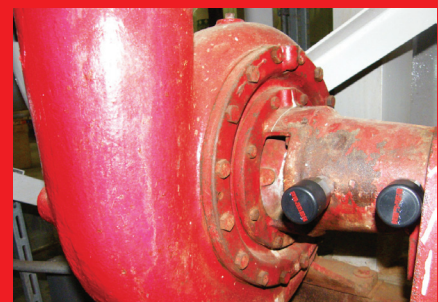
Figure 3. Ranger Sensors mounted on Talecris machinery
