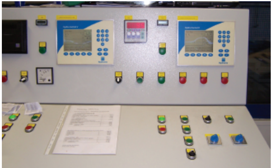
Microwave moisture measurement system installed in a plant control panel
