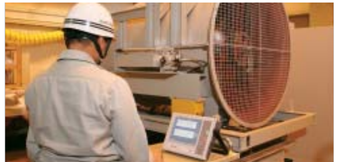
Rotational vibration measurement of a large blower using the CF-7200
