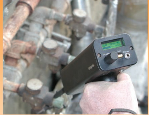
Inspect steam traps
